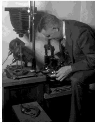
Wilmer Souder is seen using an early comparison microscope to compare the rifling marks left on two bullets, a technique for determining whether the bullets were fired from the same gun. This technique for comparing bullets is still used today in much the same way. Credit: Photo by NBS/NIST; source: NARA
